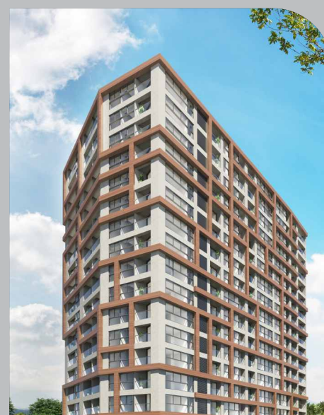
EDIFICIO LOOK AND FEEL SURCO
